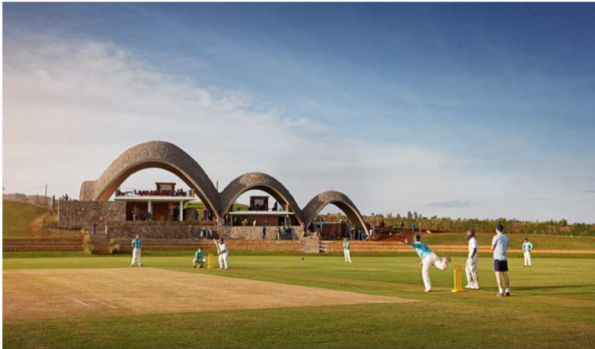
Project: Rwanda Cricket Stadium Award: 2018 Structural Award for small projects of under 1 million
